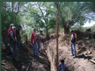
Local high school students helping with the construction. February 2005.
