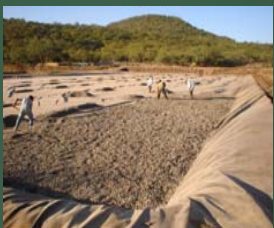
Workers spreading the filter media in cell #1. May 2005.
